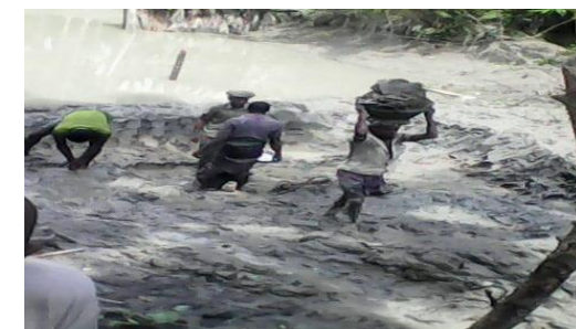
The work of road repairing is going on by the WCC
