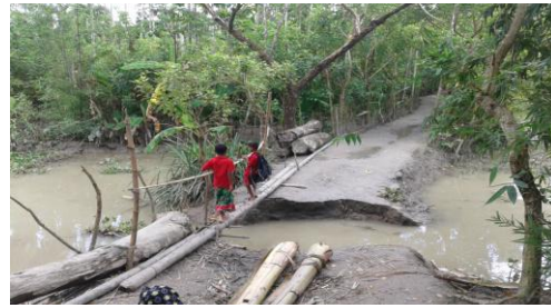
A serious problem of people by the broken road
