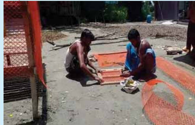
Photo: For beneficiaries, scaffolding is being prepared Photo credit: COAST Date: 15/09/2020
