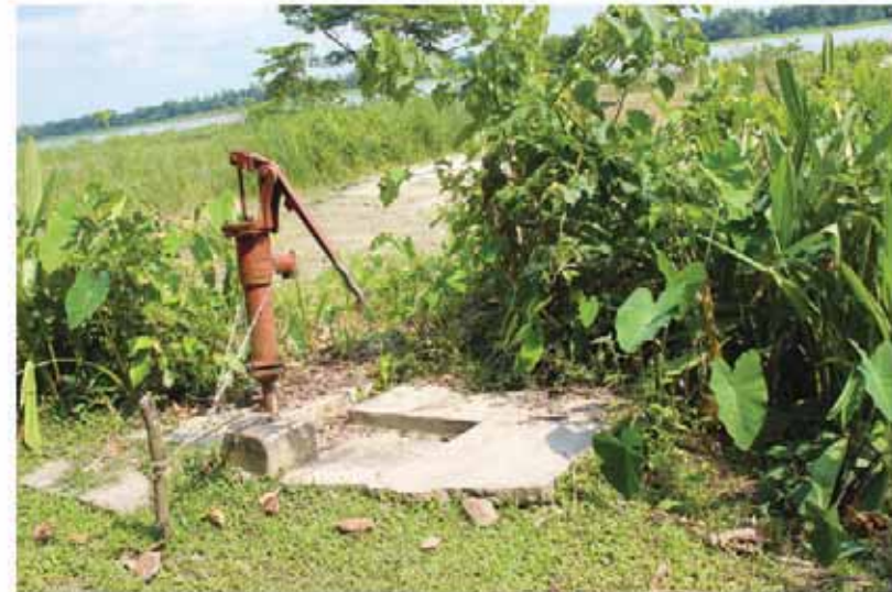
According to the Union Parishad and locals, the groundwater level has dropped by almost 60-70 feet in the last 15 years, around 30-35% of the 800-900 feet deep tube wells are completely unusable. Credit: 6 no-Ward, Central Jainkathi, Patuakhali.
