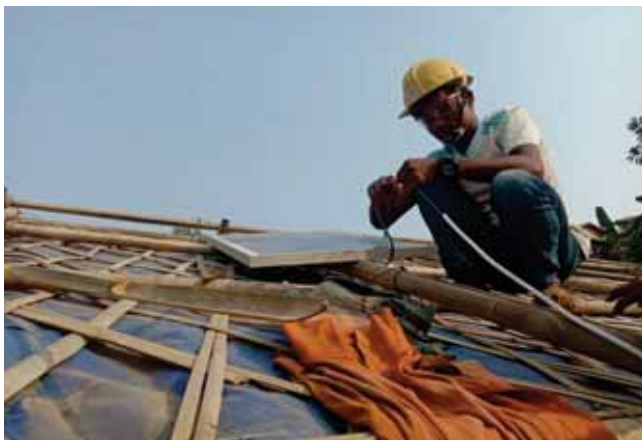
Jamil is busy in repairing solar panel at neighboring house. Photo- Selina Akter, SW
