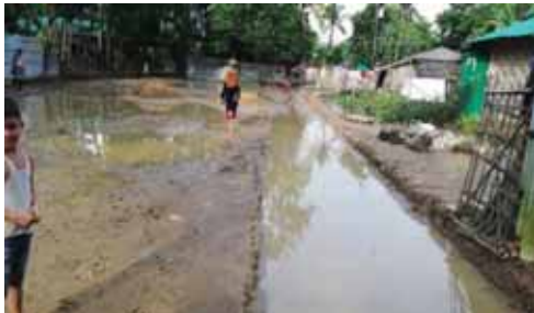
Road of Hoakbrang before construction. PC-Feroja
